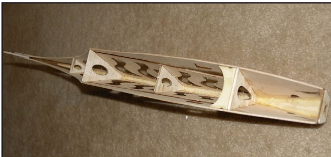
Assemble and glue back (spine) lite-ply piece to body. Some sanding will be required for a good fit. Then glue front motor mount to face with epoxy. Glue lower body pieces in place. Sand battery hatch for a good fit.
